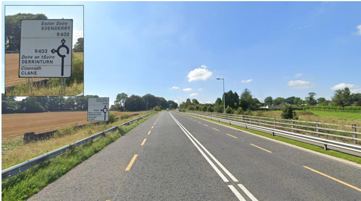
Plate 14-5: R402 Southbound at R402/R403 Junction Source: Google Street View Aug 2021
