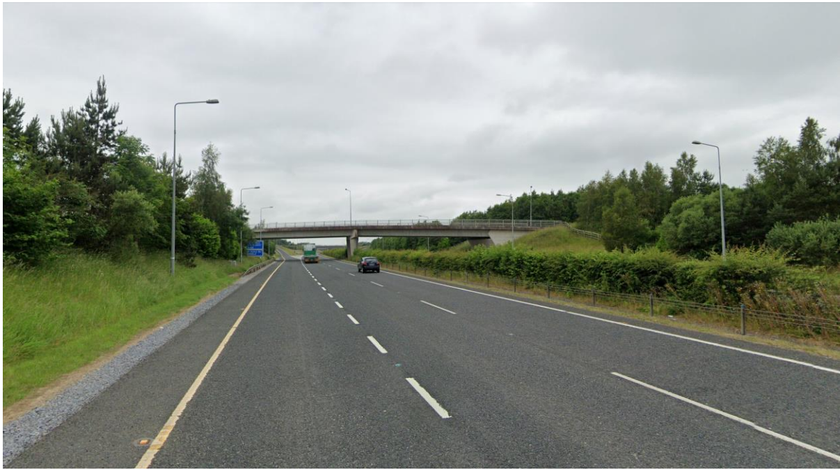
Plate 14-3: M4 Motorway Westbound between J8-J9 Source: Google Street View Jul 2021
