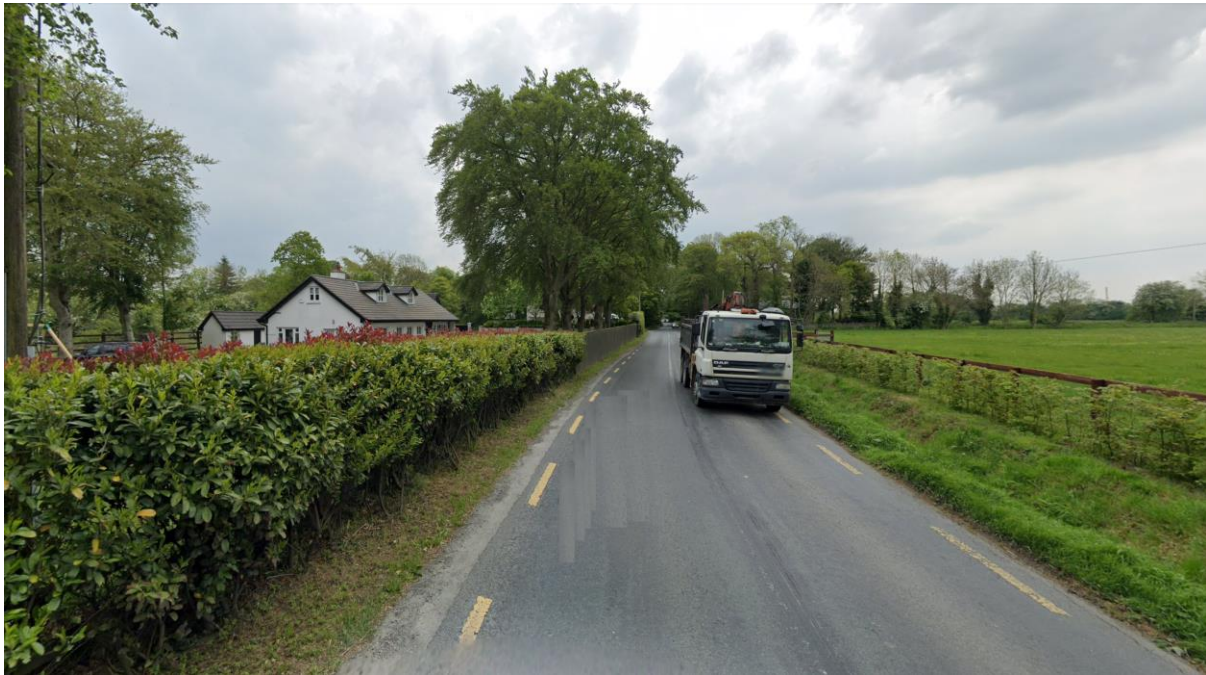
Plate 14-12: L2002 Northbound Approx. 1 km North of R407 Source: Google Street View May 2019
